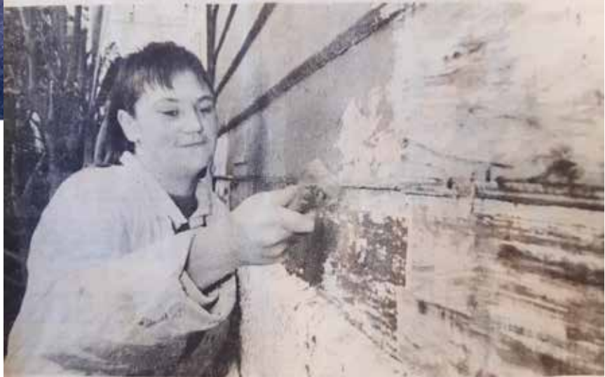
Top Otago apprentice painter and decorator Sharlene Pepper removes the old paint from this Somerville Street residence in preparation for a new coat.
