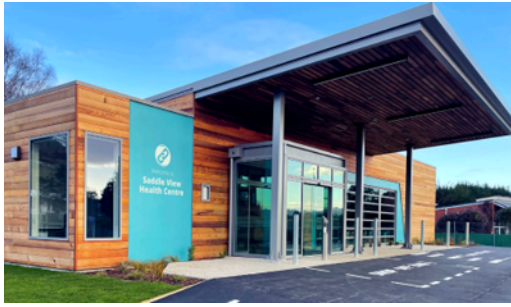
Saddle View Medical Centre: 242 Main South Road, Green Island
