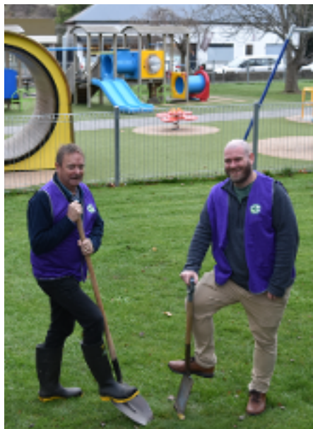
Steve Hayward and Ben McKenzie break ground for the Stage and BBQ.
