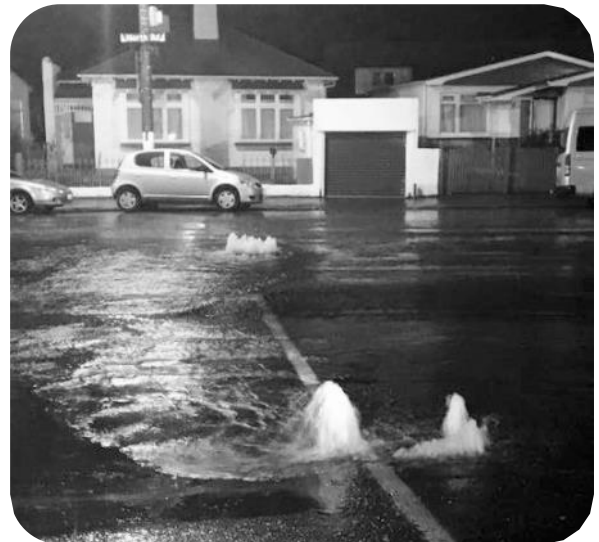
Manholes on James St pop up as water overflows from the stormwater pipes during flooding this July.
