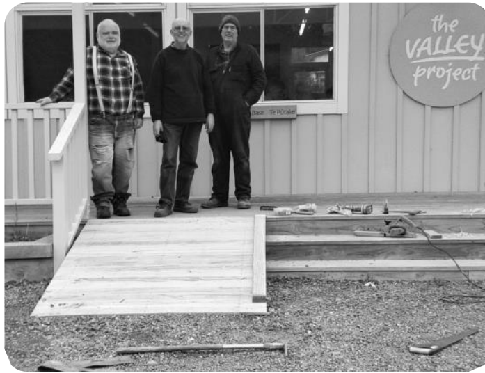
Disabled access to the Valley Project community rooms, or for anybody pushing a pram, is now a lot easier with a wider ramp which was made and installed by members of the North Dunedin Shed. Pictured installing the ramp are, from left, Gerard Kenny, Paul Nelson and Wayne Jefcoate.
