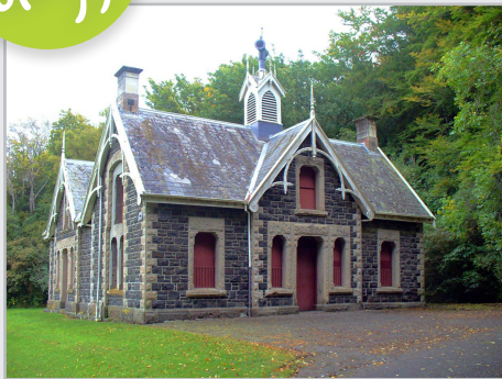
The old roof on Chingford stables, replaced in 2020. Photo: Shelley Morris
