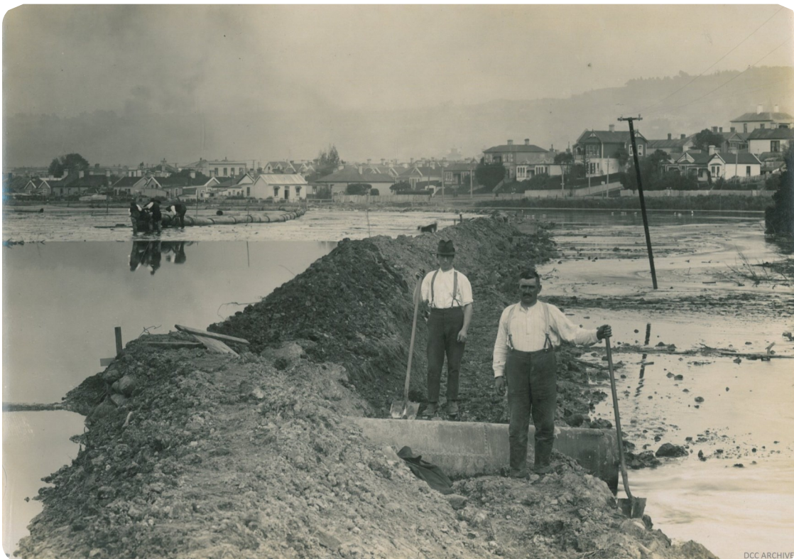
Early work on reclaimed Pelichet Bay for building work. Taken some time in 1924.
