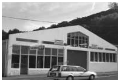
The Allen Street building
