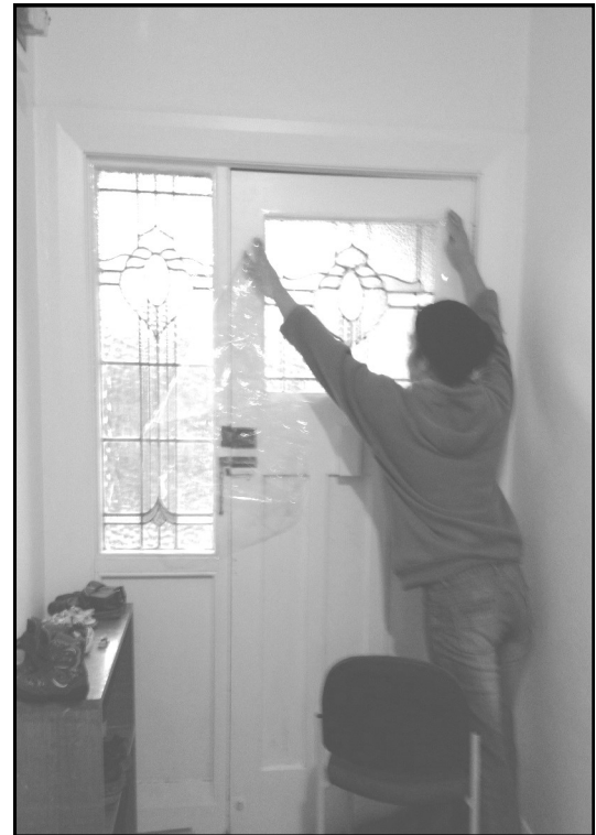
The Cosy Home Flash Mob in action. Chris Rogers prepares double insulation film to go over windows. Anau Fasita installs window film over the glass of a front door.
