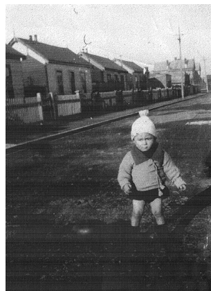
Houses in Waverley Street, South Dunedin. The first house Joseph and Wurrdi owned in their street would have been identical to the ones shown here.
